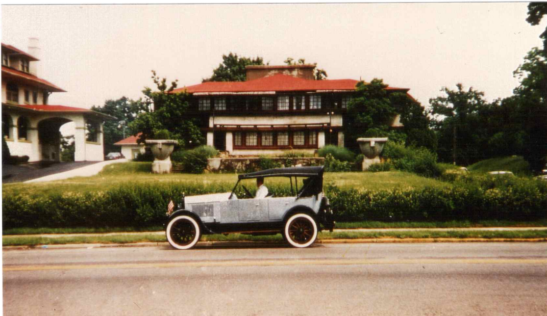
WESTCOTT HOME IN SPRINGFIELD, OHIO WITH A WESTCOTT CAR IN FRONT OF IT.
